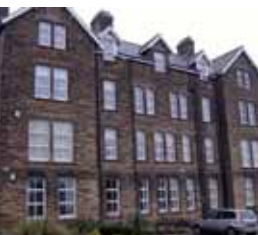
South-West Front Cavendish Mill
