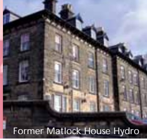
Former Matlock House Hydro
