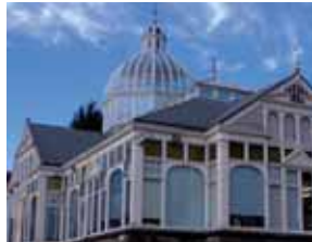
Former Winter Gardens Smedley's Hydro
