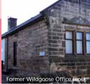
Former Wildgoose Office Block
