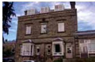
Former Bank House Hydro
