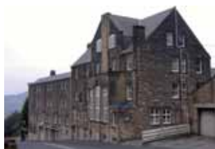
Former Chatsworth Hydro
