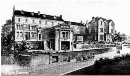
Oldham House and Prospect Place Hydro postmarked 1912 Point 29a/29b
