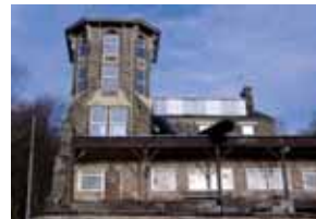
Former Jackson House Hydro
