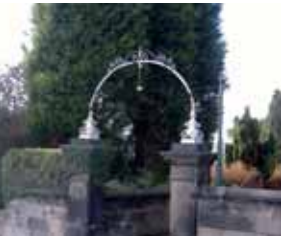
Pedestrian Entrance from Chesterfield Road, Former Chatsworth Hydro
