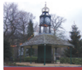
The Former Tram Shelter
