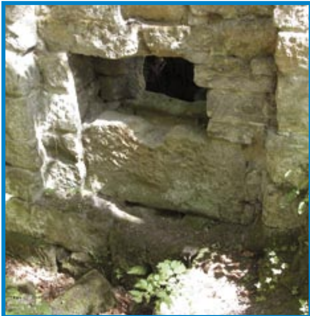
Detail of the stone which held the axle of the waterwheel at the Paint Mill
